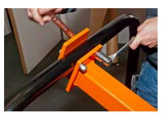
8. Fit the sliding rail. Start by fitting it to the tube arch using **two M10x80 + M10 lock nuts** and **M10 washers** on the side where the nuts is.
